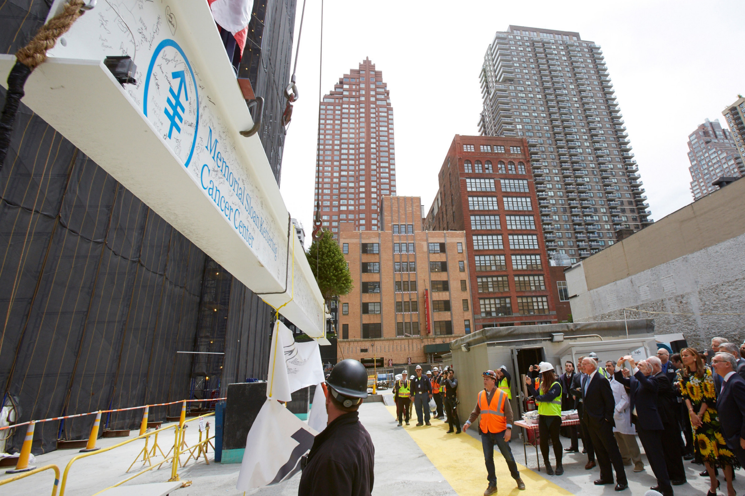
MSK's David H. Koch Center for Cancer Care under construction
